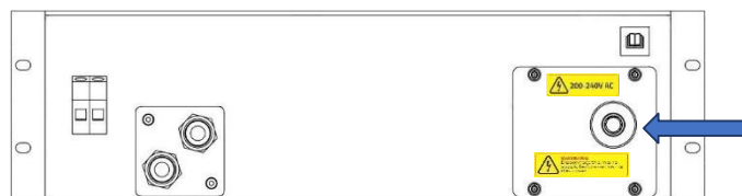
Figure 59 - AC power connection point
